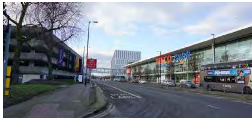
Queensmere multi-storey car park and Tesco superstore on Wellington Street
