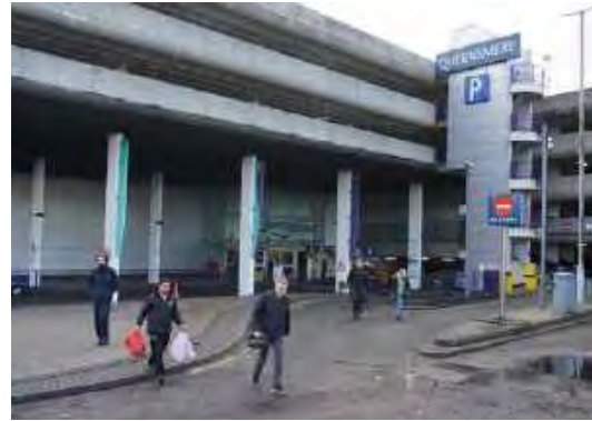
Inhospitable walking environment at the entrance to the Queensmere Centre on Wellington Street
