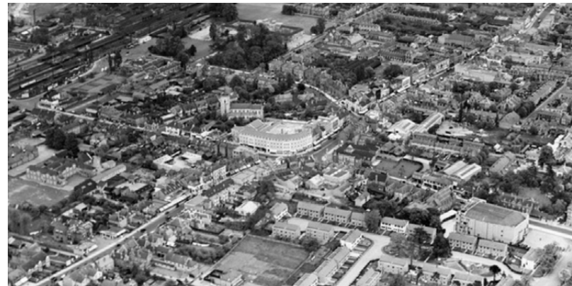
Aerial view of Slough town centre from the south west (circa 1930) © Britain from the Air
