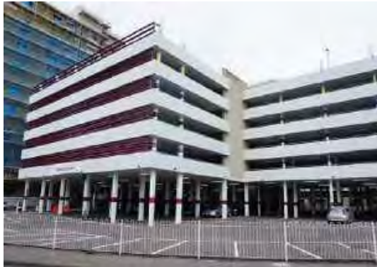
Hatfield car park has been recently refurbished
